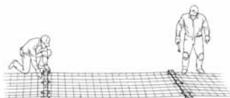
1) Position the Stretcher Bars under the Fence
