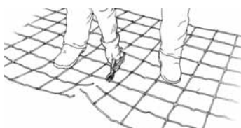
4) Cut the Line Wires Between the Stretcher Bars
