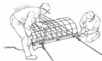
8) Crank the Puller Handle to Tighten the Fence
